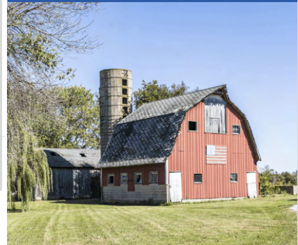
Partially Enclosed Building
